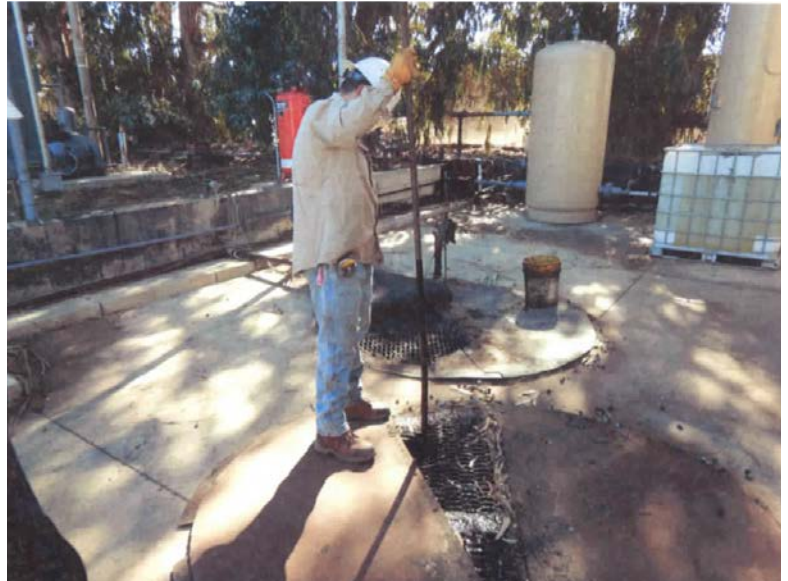
Figure 7. Metal-Lined Tank – Oxnard (CFROG 2016)
