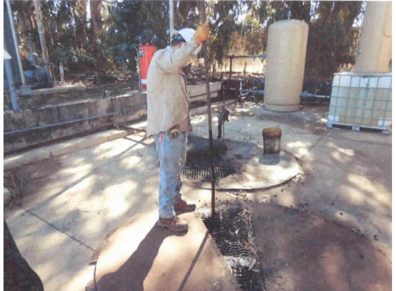
Figure 7. Metal-Lined Tank – Oxnard (CFROG 2016)
